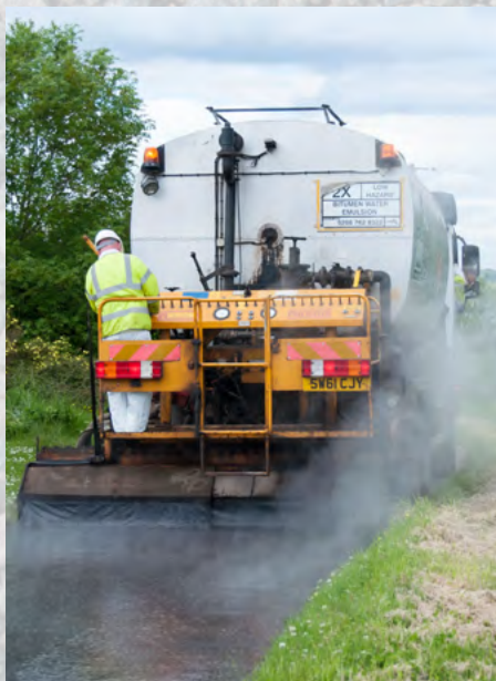
The road surface is sprayed with bitumen emulsion
