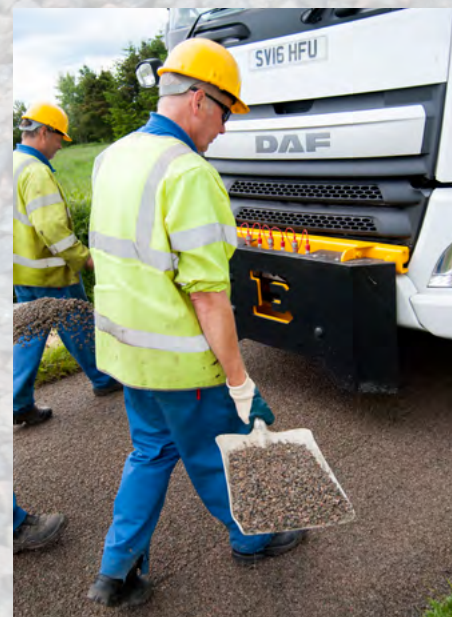
Inspecting and patching any parts that are missed is done by hand
