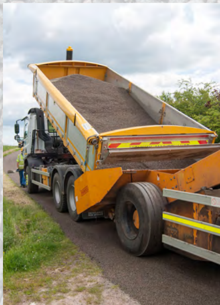
Loading the hopper, while the spreader is still moving forward
