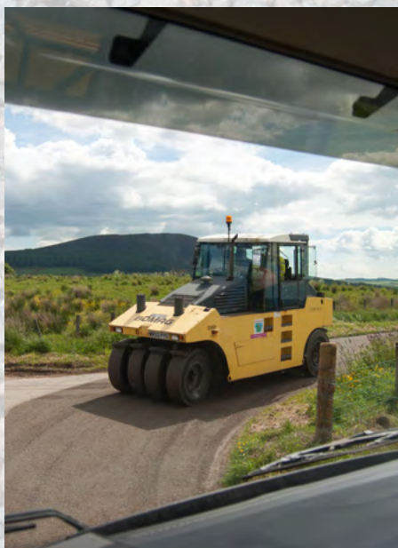
The roller helps to bed the chippings into the emulsion
